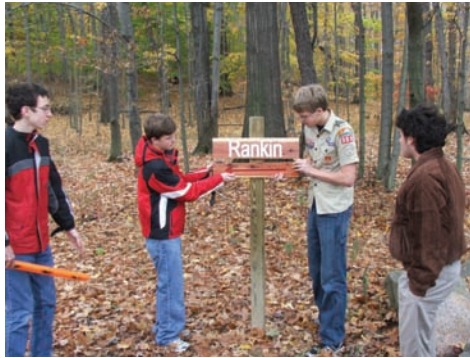
The finished product. Wilson and friends from Troop/Crew 309 install the markers which will help residents navigate our trails.
